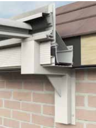
Custom designed gallows brackets are sometimes required
